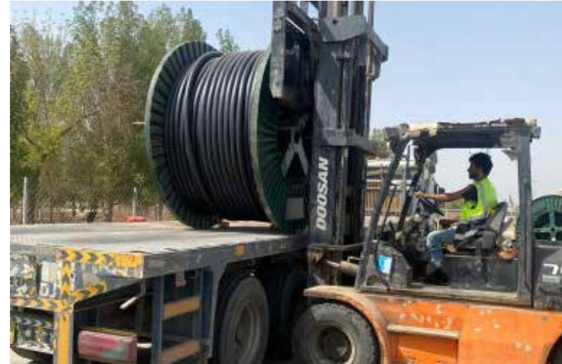
▶ Pulling cables in meter: 41,584
