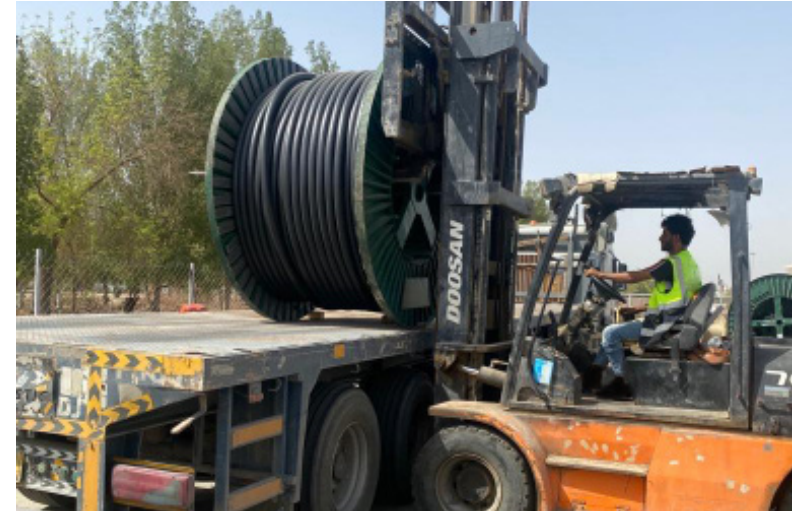
▶ Pulling cables in meter: 41,584
