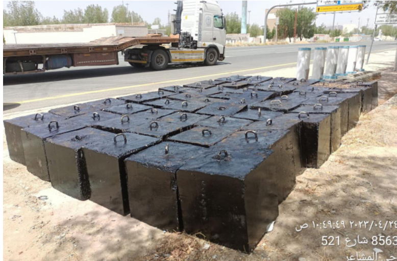
▶ Concrete foundation for tents, number: 1,296
